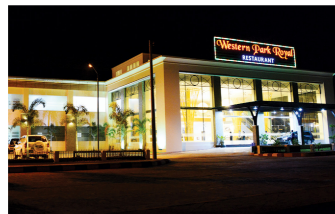
Western Park Royal Restaurant Location: Nay Pyi Daw Lift: 2 units of Escalator
