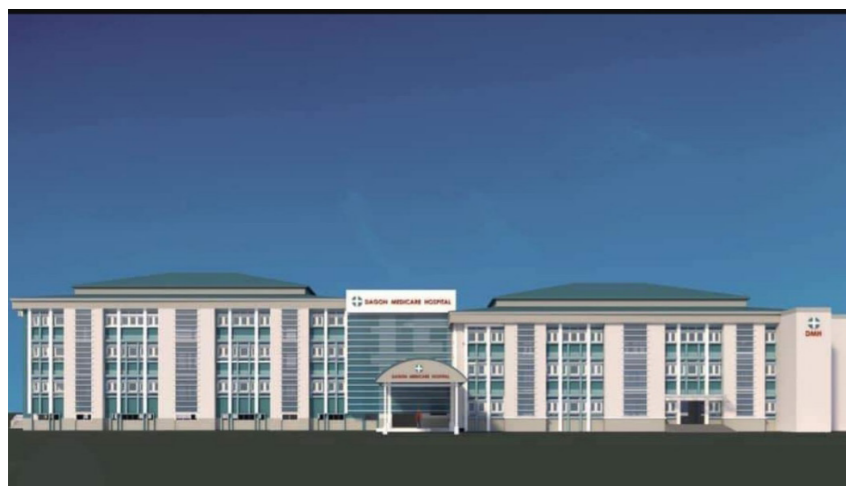
Dagon Medicare Hospital Location: Yangon Lift: Total 7 units of Bed Lift 1 unit of 1350 kg- 3 stops 3 units of 1600 kg- 3 stops 3 units of Hydraulic vertical bed lift- 3 stops
